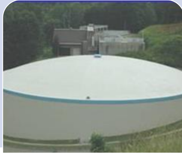
Concrete Tank Coating
